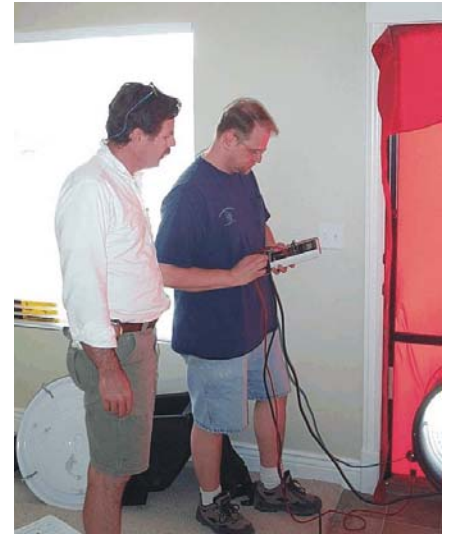
Energy Rater performs blower door test to measure air tightness.
