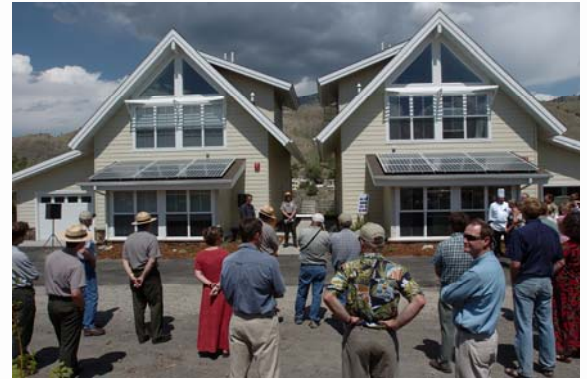
LEED Certified residential units at Yellowstone National Park in Yellowstone, Montana built using an ICF system.
